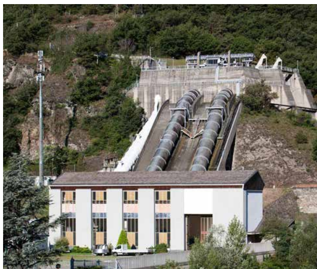
Montjovet power plant
