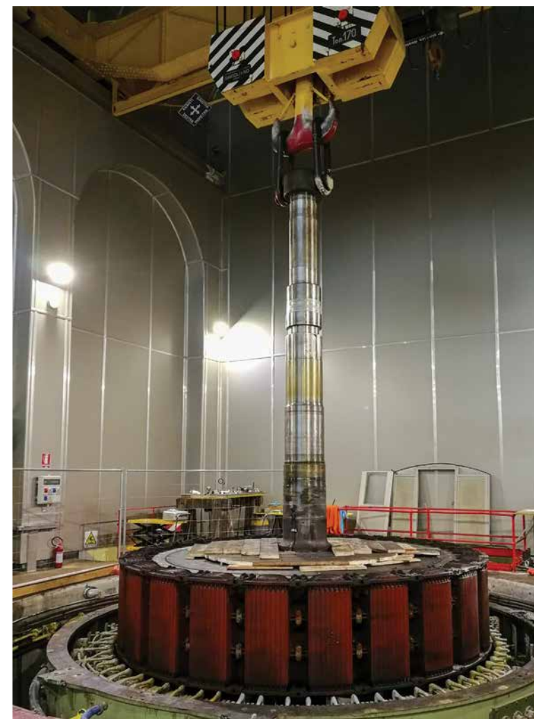
Rotor extraction of the Hône 1 power plant
